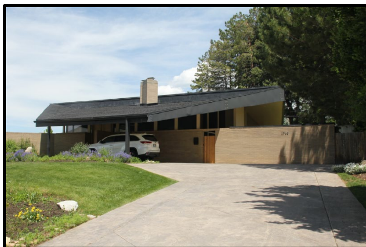
Southwest elevation of house, facing northeast – 2020.
